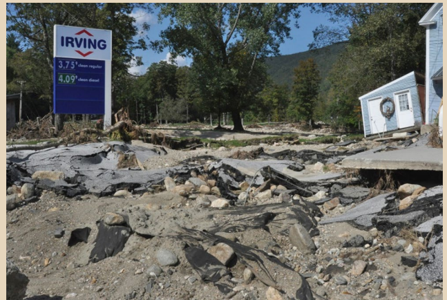
Blackie's General Store - Soil erosion and scour from Ottaquehee River flooding. Tropical Storm Irene - August 2011. Credit: New England Interstate Water Pollution Control Commission
