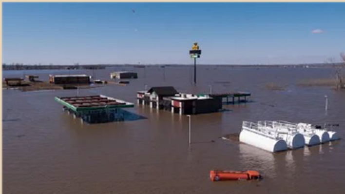
Flooded gas station with USTs and ASTs. Credit: EPA
