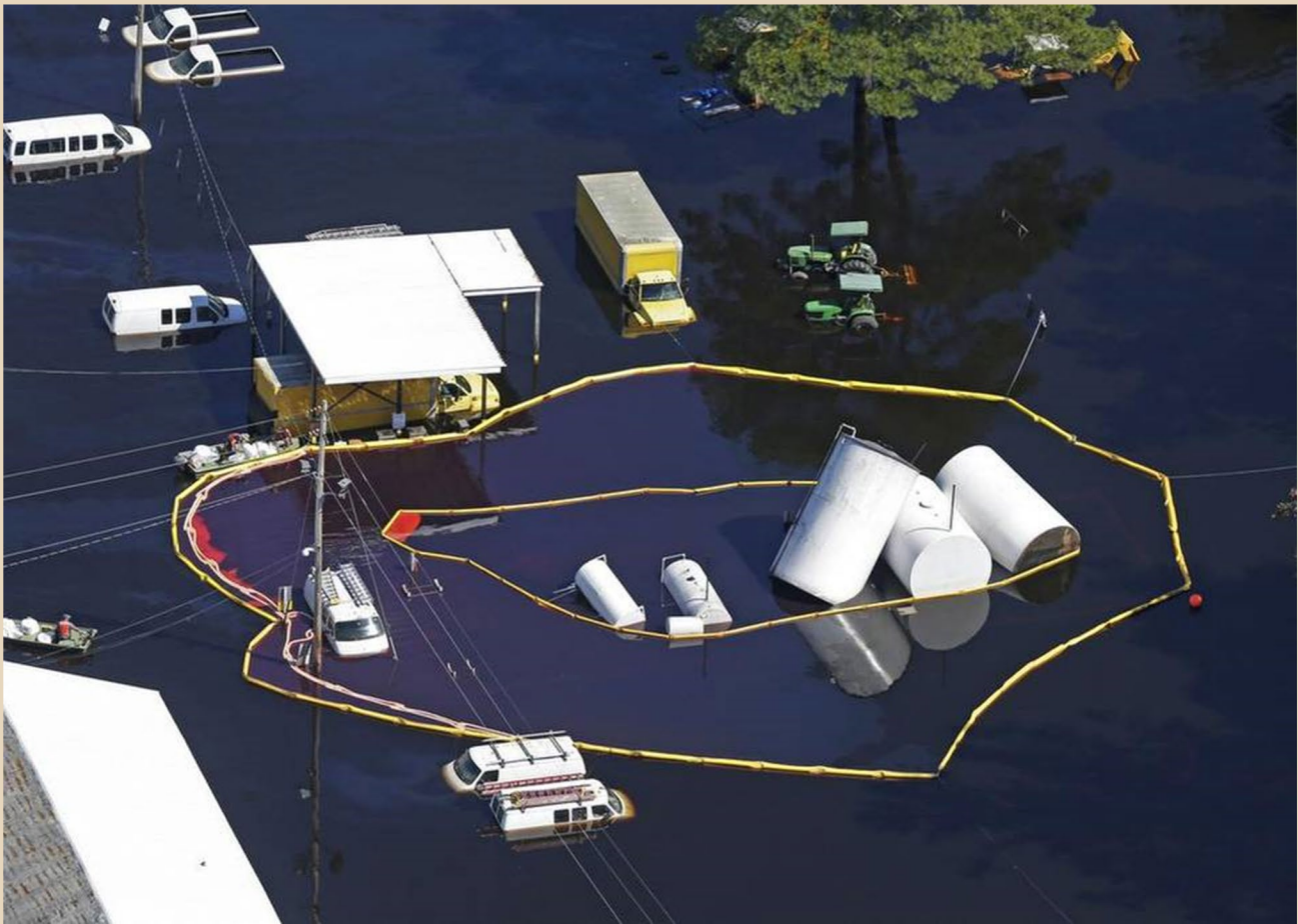
Facility with displaced ASTs, product release, and fuel containment – Hurricane Matthew, 2018. Credit: NCDEQ
