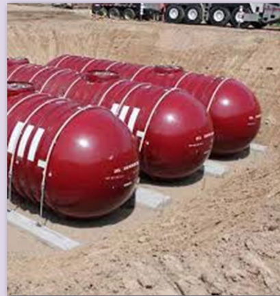
UST deadmen installation. Credit: ZCL Composites
